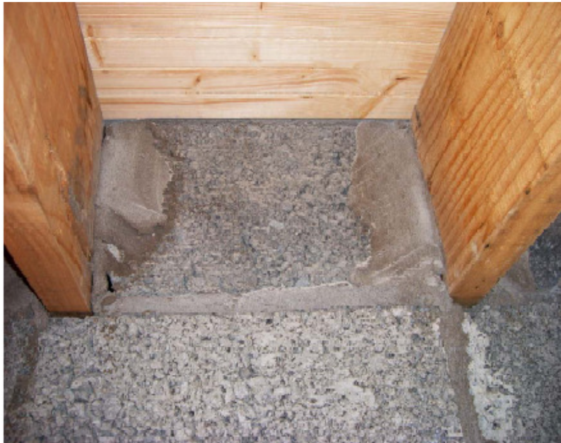
Sealing at intermediate floors: First stage: point up around joists
