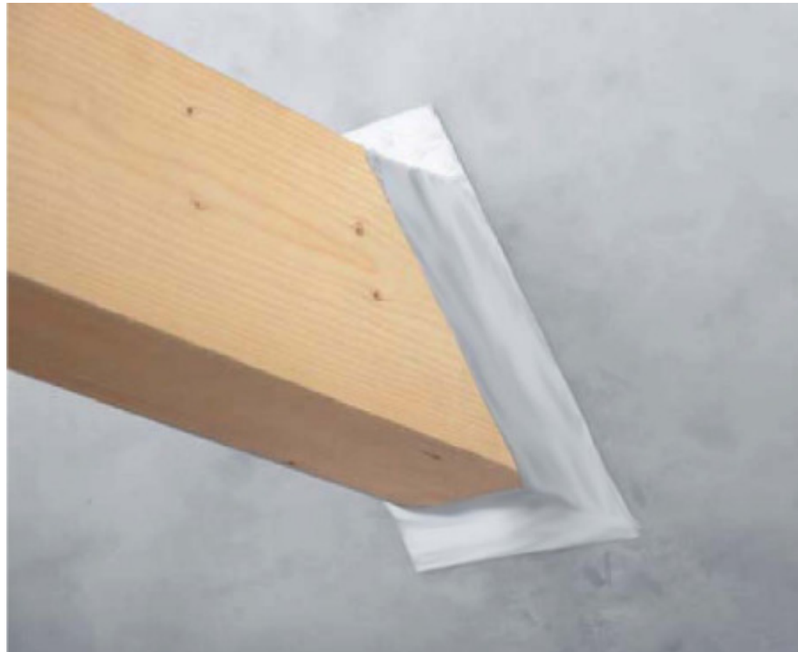
Sealing the junction between the joist and the external wall
